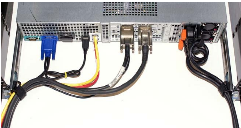
Figure 11: Cabling a System Installed in Static Rails
